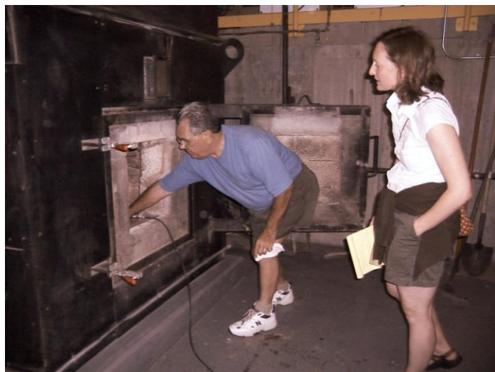
Cusack peers into the Mt. Abe boiler.
